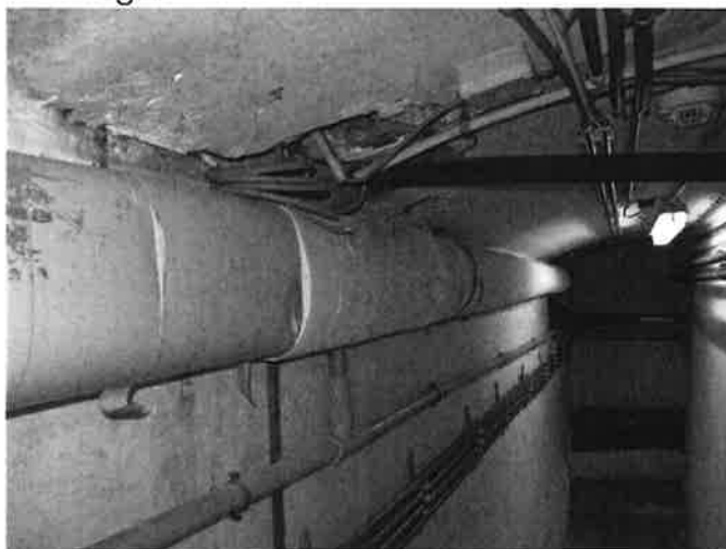
Photo 1+2 PASCAE -1.12 couloir cave calorifugeage plâtre + isolant
